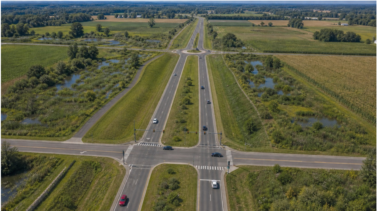
Figure 5. Photorealistic visualization of the Greenway's landscape and access strategy. The divided roadway, protected landscape, separated path, surface-water system, and selected at-grade junction illustrate the project's integrated design. Intersection forms are alternatives selected by context rather than a fixed consecutive sequence.
