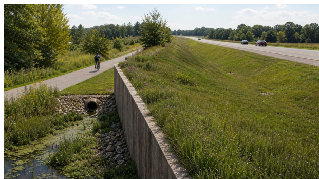
Figure 6. The landscape-facing “Ha-Ha” boundary. The abrupt face belongs on the landscape and trail side; the road side rises as a gradual landform toward the Greenway roadway.
